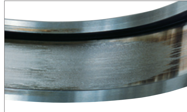
Photo 7-4-2 Part: Outer ring of Photo 7-4-1 Symptom: Smearing occurs circumferentially on raceway surface Cause: Roller slipping due to excessive grease filling
