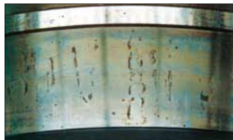
Rust and corrosion
